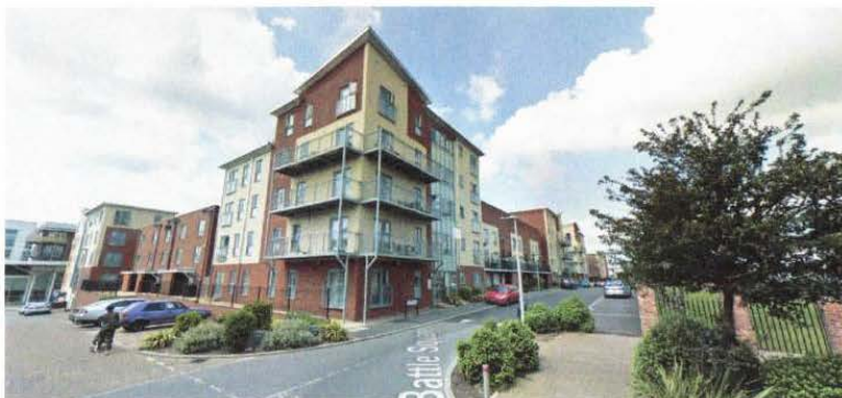
Curzon Street/Battle Square residential development 200m east of Grovelands Chapel featuring large balconies and windows facing the main road
